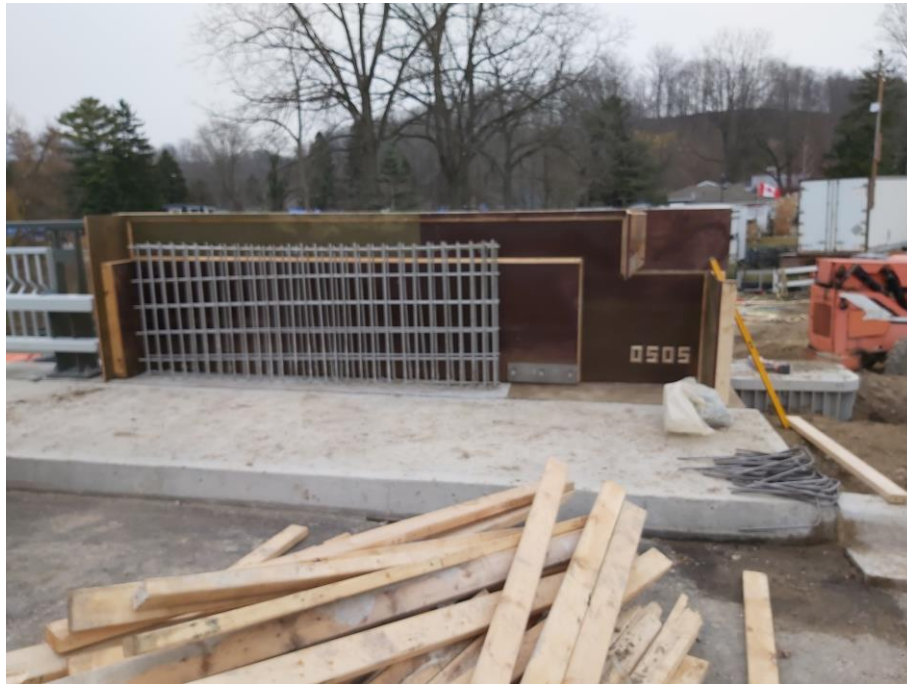
Photo 1: South end post partial formwork and reinforcing steel installation
