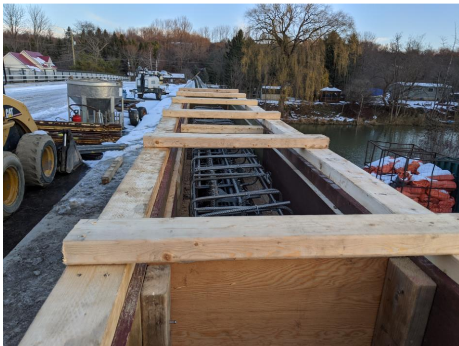
Photo 2: South end post formwork 'closed-in'
