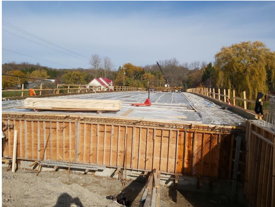
Figure 3: The bridge deck curing under vapour barrier
