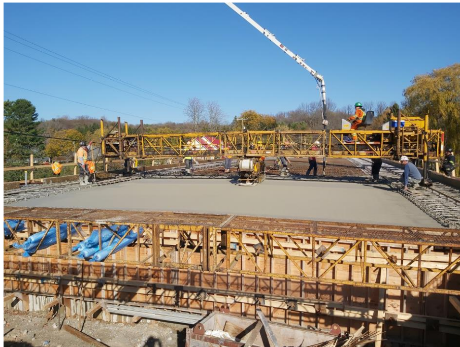
Figure 2: Bridge deck pour in progress
