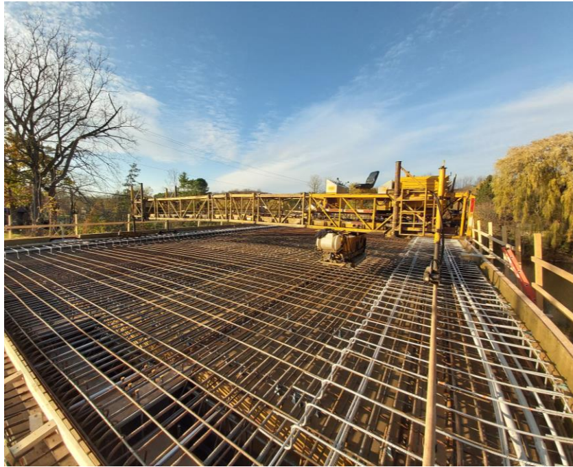
Figure 1: Bidwell set up in anticipation of the bridge deck pour
