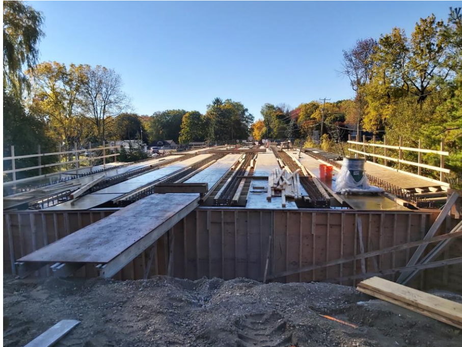
Figure 1: Deck falsework installation
