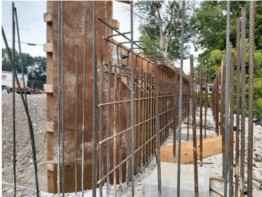
Figure 1: Rebar installed on the south abutment
