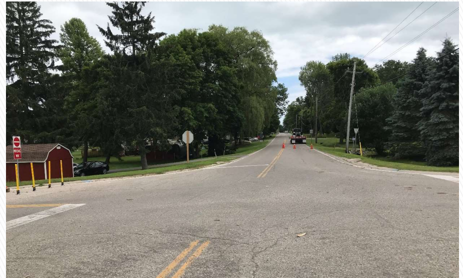
South Approach (looking south)
