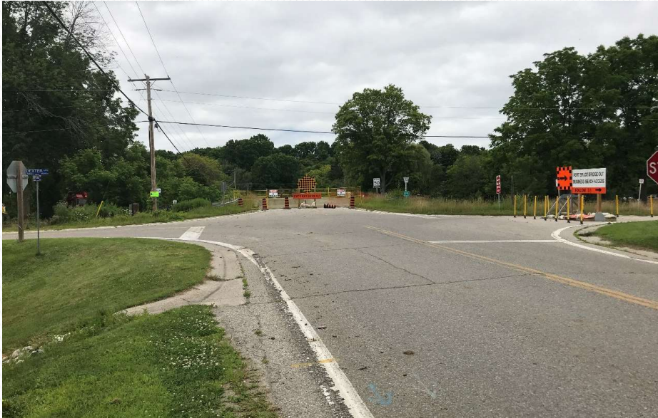
Far South Approach (looking north)
