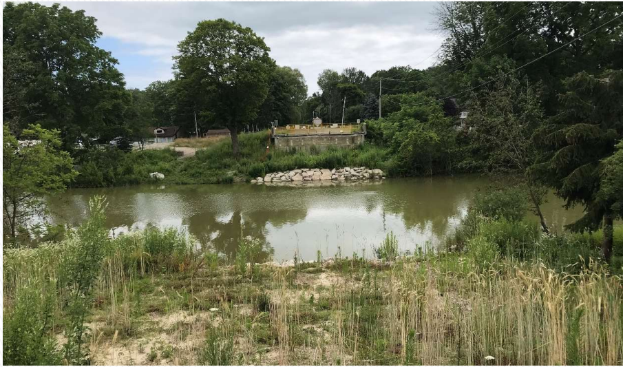
North Approach (looking south)
