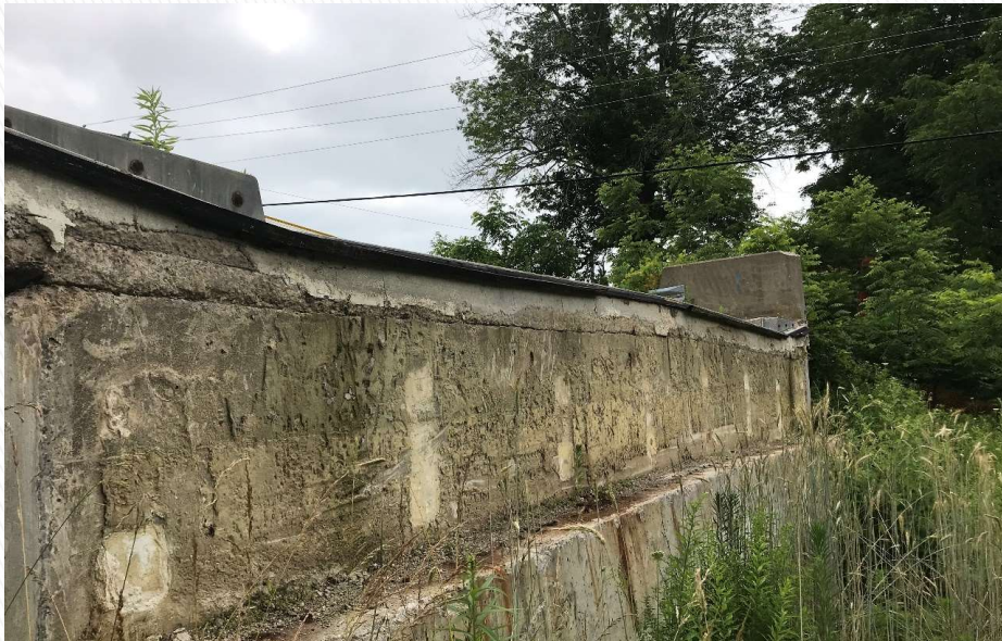
Existing South Abutment
