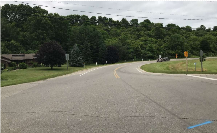
North Approach (looking north)
