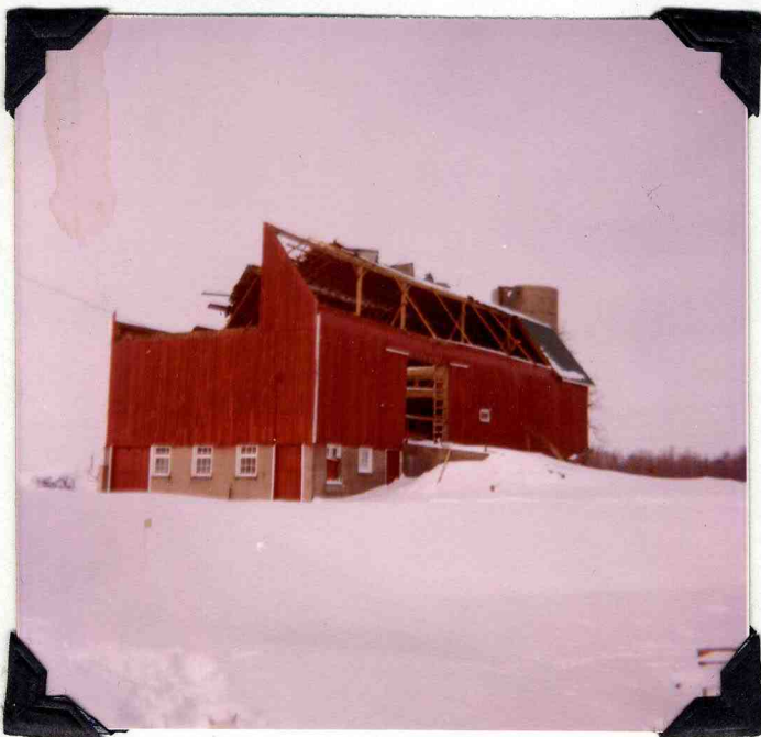
Clayton Reid's barn 10th conc. Upper structure and roof damaged.
