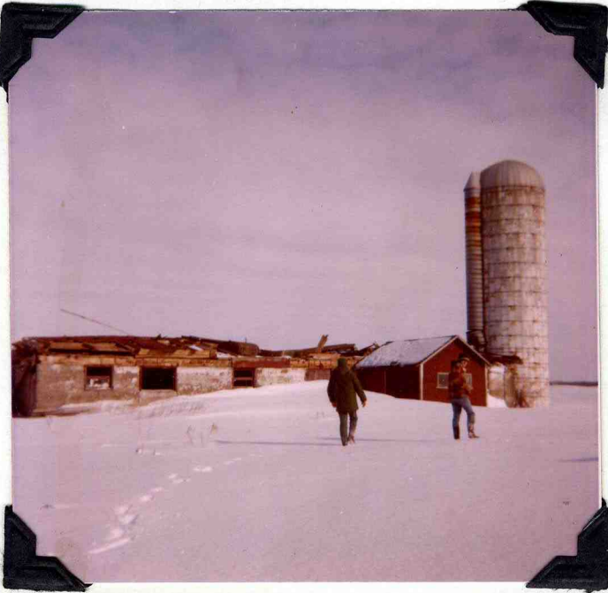
Clayton Reid's barn Edgware Road Completely demolished
