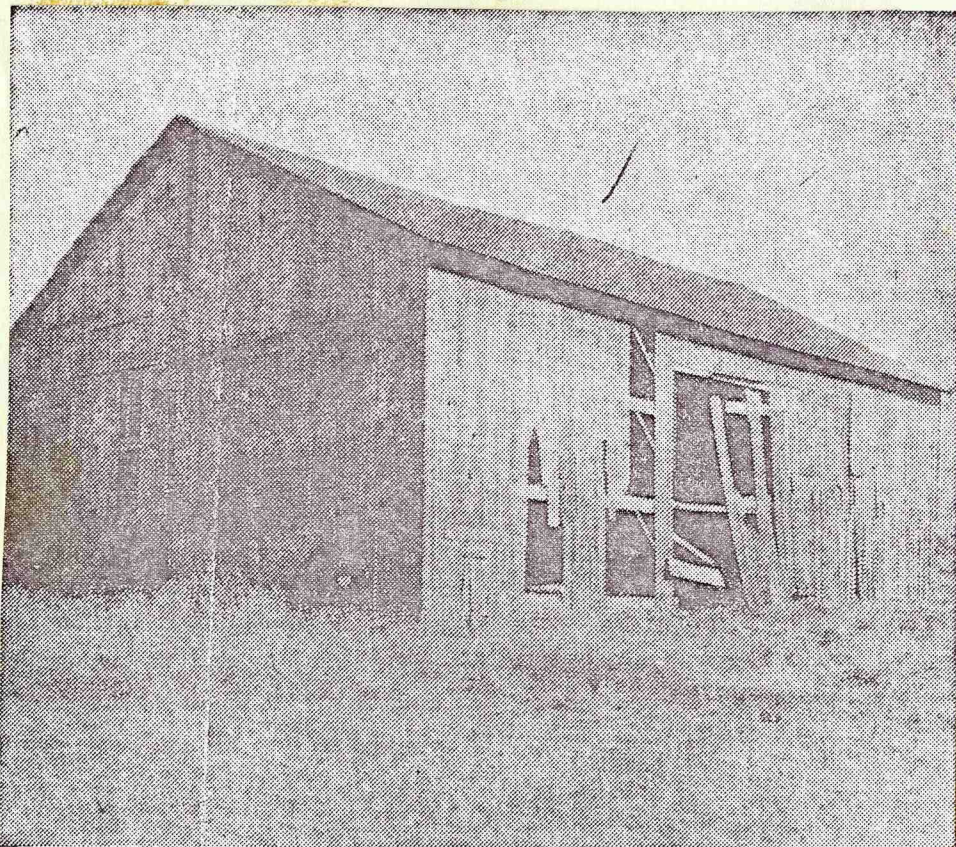
Demolished some time ago, this barn on the former Sinclair farm was the last remaining building in the Locke's Springs vicinity. The farm is now owned by Donald Burgess.
