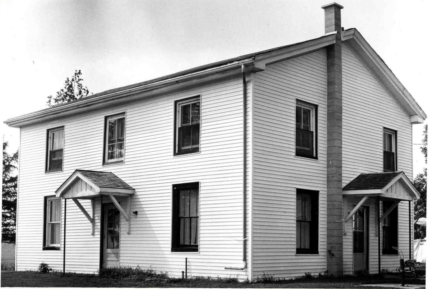
2. Although it is hard to tell from this picture this home, owned by Mr. and Mrs. Keith Davis at R. R. 8 St. Thomas, was the first brick house in North Yarmouth township. The large structure was constructed by Duncan McGregor, an early Scottish emigrant, possibly as early as 1840. The home is located on Elgin County Road 52 and has now been covered with siding.
