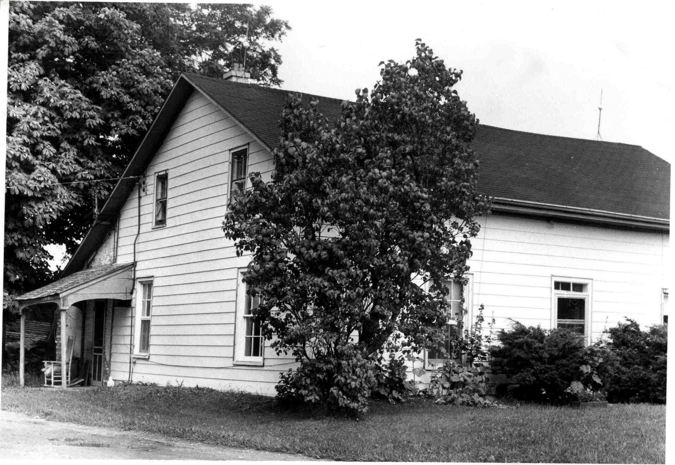
1. The home of Mr. and Mrs. Calvin Watson on County Road 52 at Radio Road is a well-preserved "mud walled" or adobe home which has since been covered with aluminum siding. Built about 1850 by William Baker it is one of two such homes in North Yarmouth.
