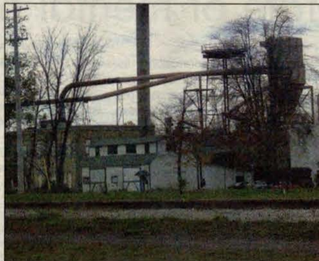
The smokestack at Erie Flooring often is seen releasing black smoke that concerns some local residents. While the plant complies with environmental controls, a new form of energy creation will help reduce emissions.
