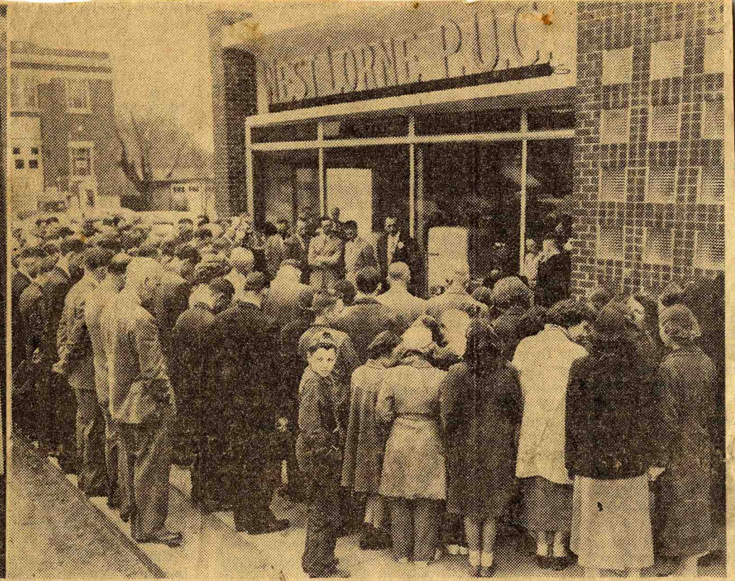
Scores thronged the sidewalk in front of the new West Lorne Public Utilities building during the ceremonies. Following the official opening by Mr. Saunders, the Rev. W. K. Morrison, rector of Grace Anglican Church, dedicated the building. Here, the crowd stands with heads bowed during the dedication. The youngster in the foreground apparently couldn't resist the temptation to sneak a peek at the photographer.
