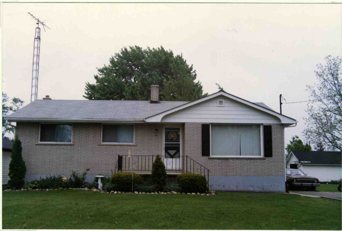
16 Argyle St. William & Jacquelin Lidster built this house in 1971
