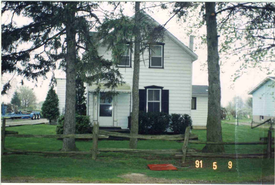
8 Queen St. owned by George + Pauline Robbins. This house is over 100 yrs. old. Originally owned by John McLean Sr. and then by John McLean Jr. Jack + Florence Lamb bought this home in 1941 and later moved to a new home at 10 Queen St.
