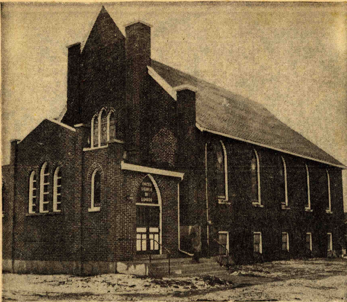
FRONT VIEW —This picture shows how a large new porchway and entrance hall has been added onto the ivy-covered brickwork of the 85-year-old
