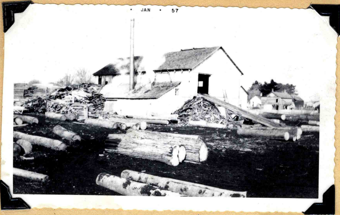
SAW MILL on Lot SOUTH EAST edge of WALLACETOWN facing north
