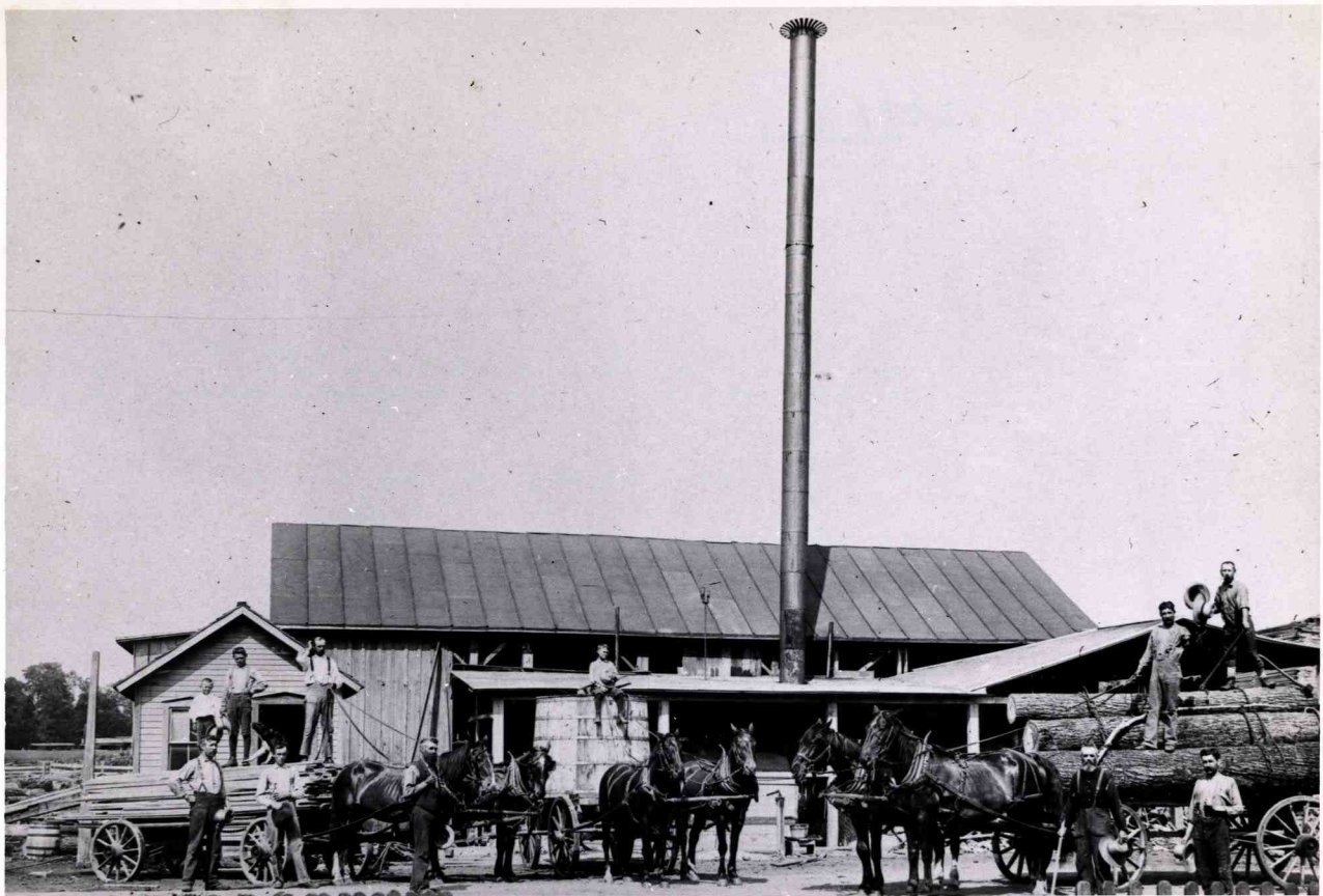
Mill built by Wm. Mobray. Later run by Wm. Plater. Rodney 1900
