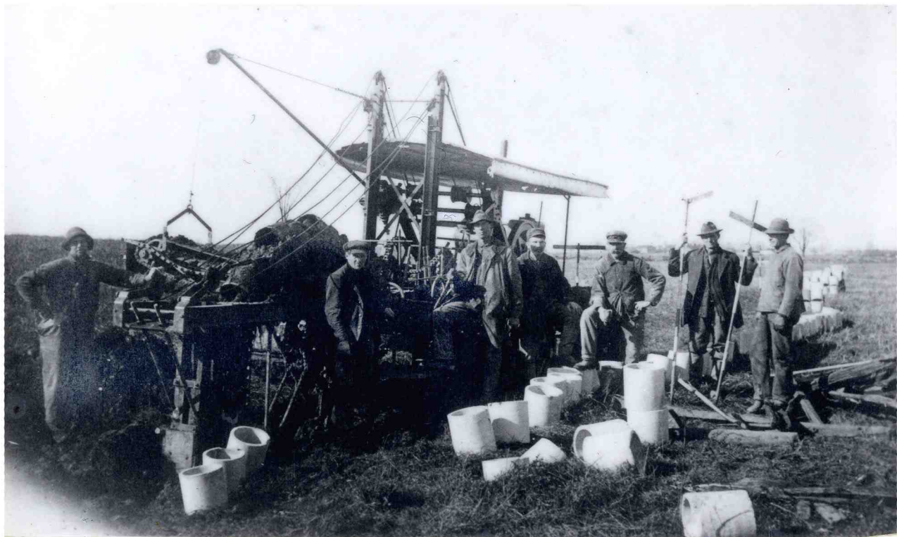
This ditching machine for laying drainage tile was owned and operated by James Reid.
