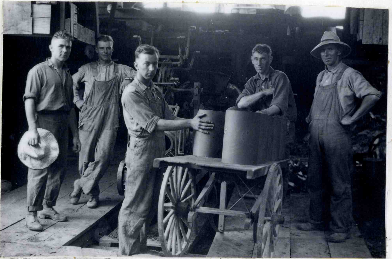
Jack Tuff, Elmore Martin, Claude Chalk, Bert Davenport, & Lorne Martin pose by a cartload of wet tile.
