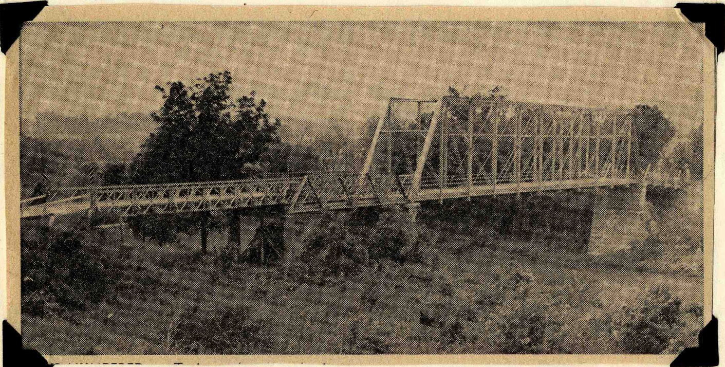
The Simpson Bridge in 1958 when a Bailey Bridge was erected to take the place of the approach which was broken when a lumber truck crashed through it.
