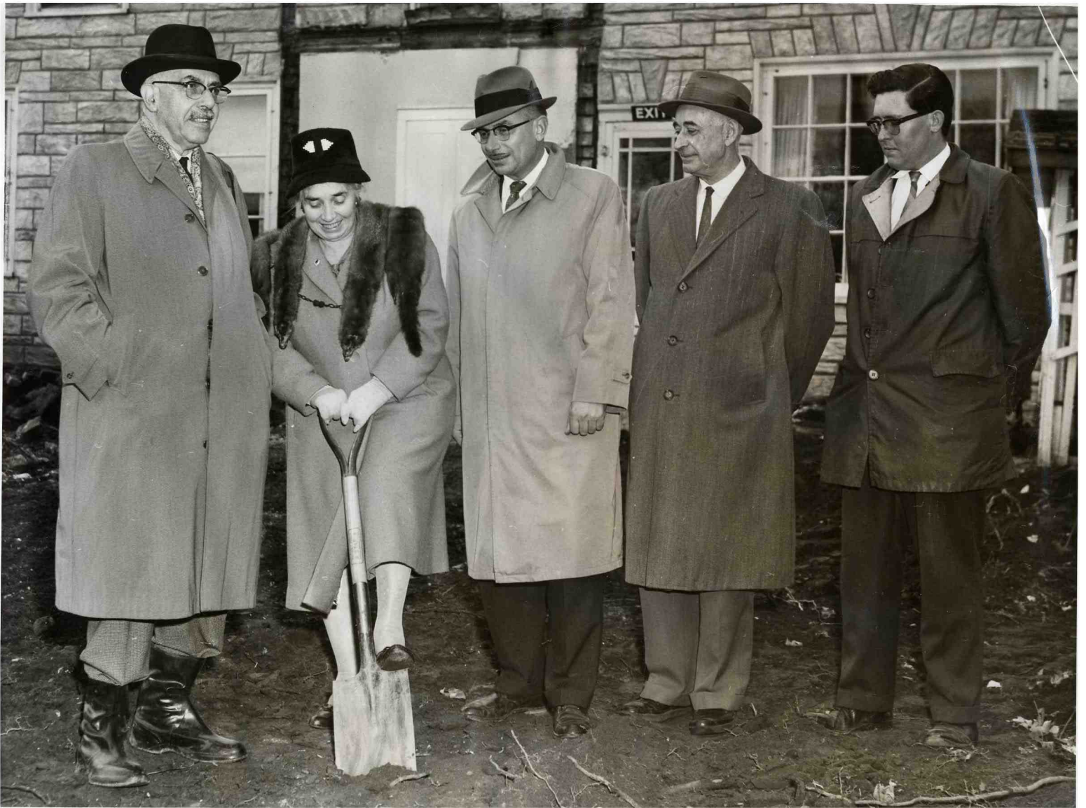
Turning Sod For Elgin County Pioneer Museum Addition Nov. 14, 1962.
