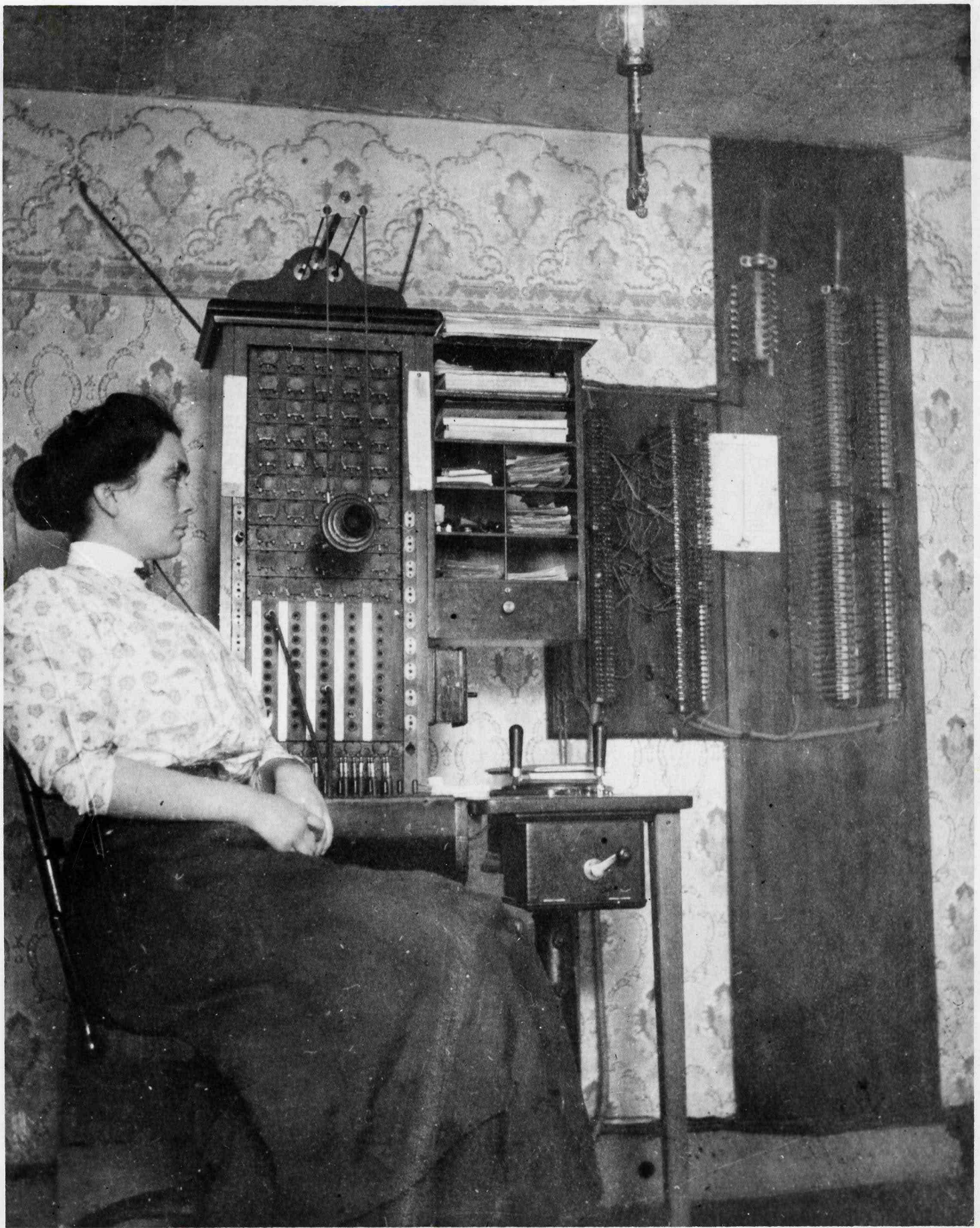
A typical telephone exchange of the nineties and early 1900's with standard switchboard and calculagraph for timing long distance calls. Belmont subscribers made long distance calls through the facilities of the Bell company by agreement with the Bell for connection with their long distance lines.
