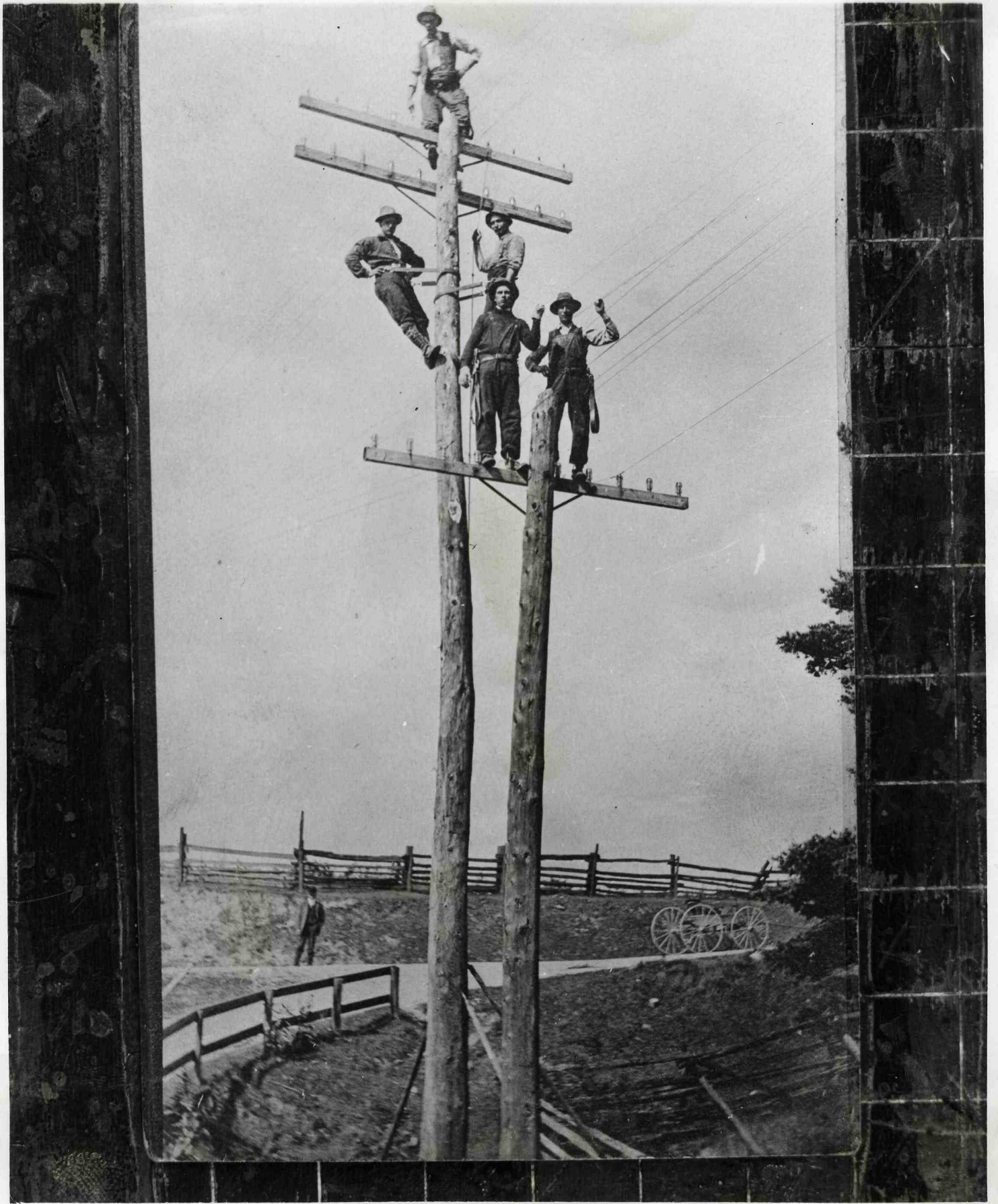
Pole line erection in the early days required sturdy shoulders and pole raising attracted audiences in town and village.
