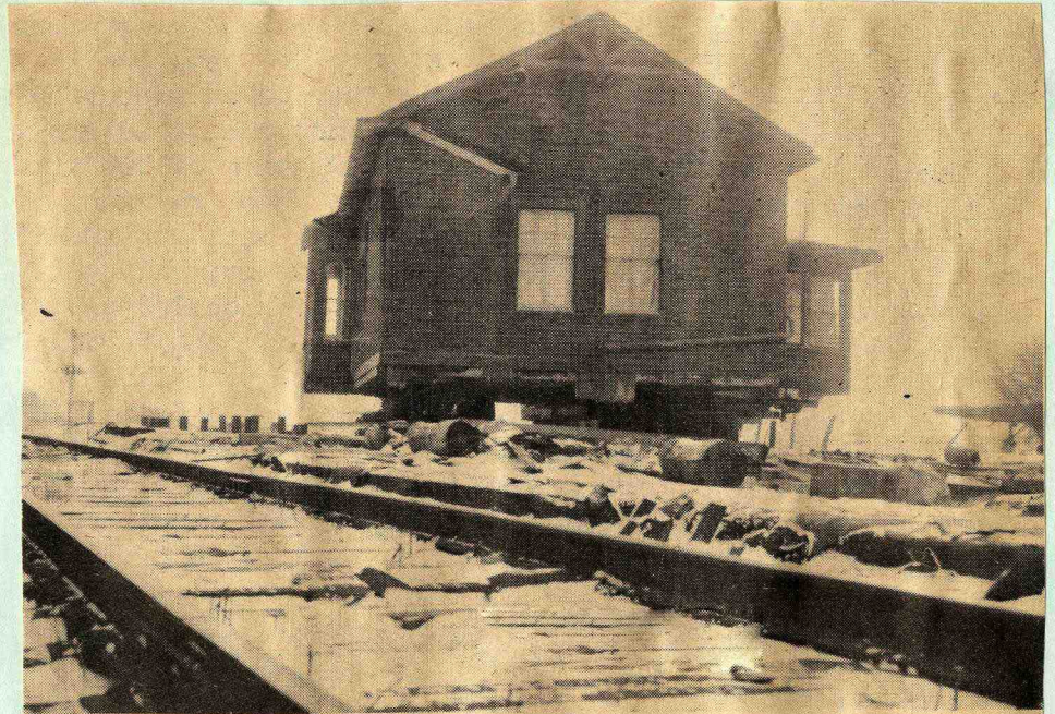
ANOTHER LANDMARK ON THE MOVE.. the old C.P.R. Station house at Belmont about to start on the trip down the #76 to a new site at Appleton. It has been hoisted up for some time and is seen here at the onset of one of Wednesday's snowstorms
