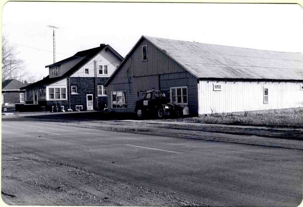
Howey Lumber office + storage warehouse
