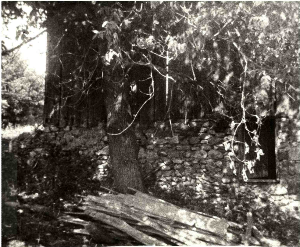
EXAMPLE OF STONE FOUNDATION FOR BARN
