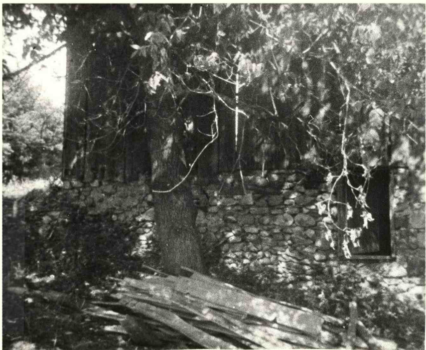
EXAMPLE OF STONE FOUNDATION FOR BARN
