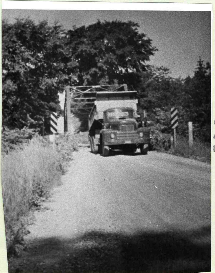
WEST ROAD BRIDGE
