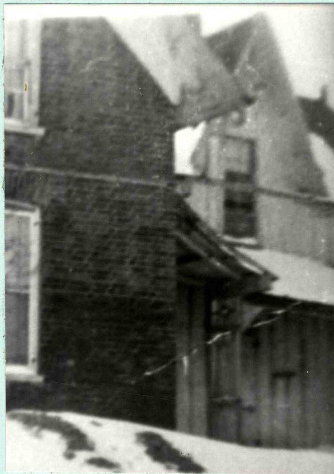
Picture showing older frame house at the back of the brick house
