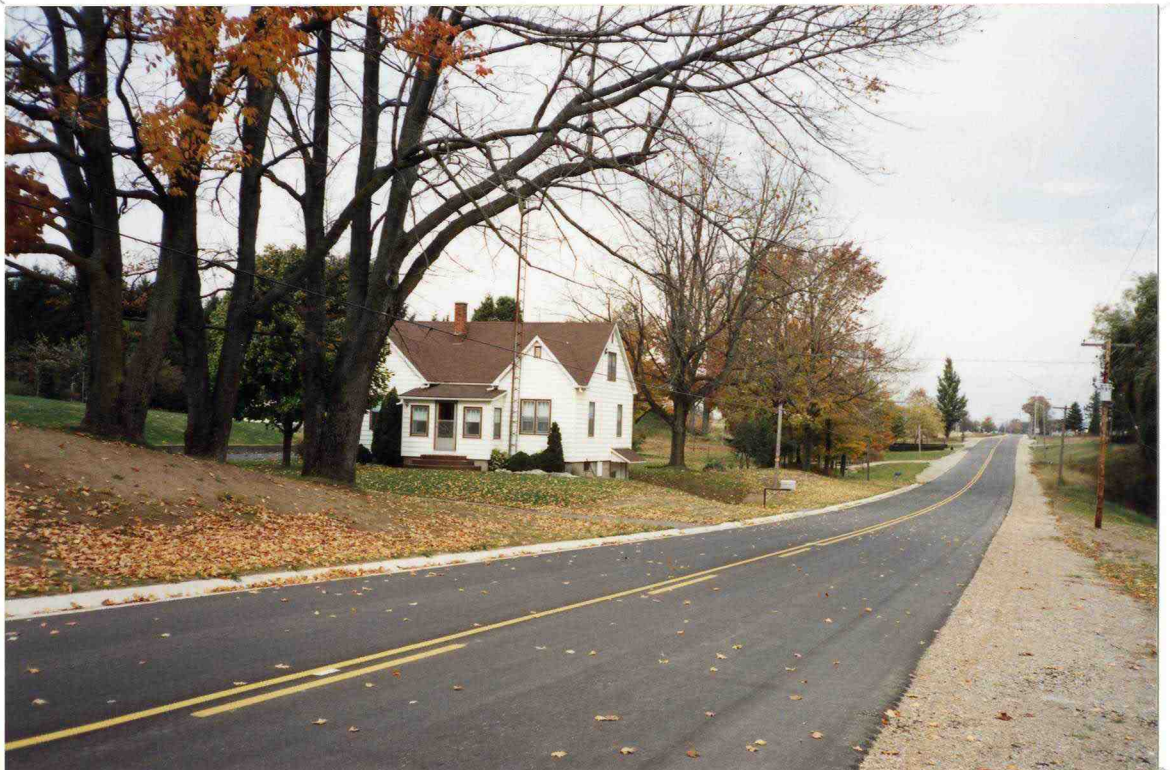
1991-05-07 COMPLETED ROAD AT WOLFE HOME
