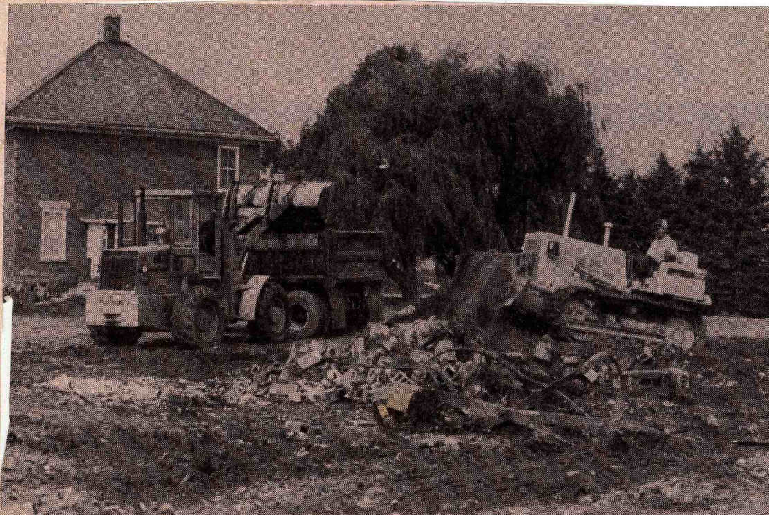
The old round barn north of Lyons was demolished by bulldozers on Friday. The 70 year-old structure was demolished and the bricks were dumped in an old irrigation pond
